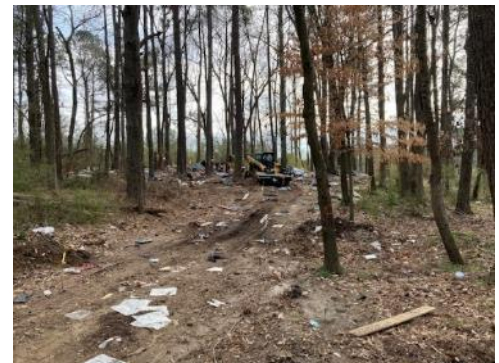
Unsafe house cleared within the Allatoona Gateway area
