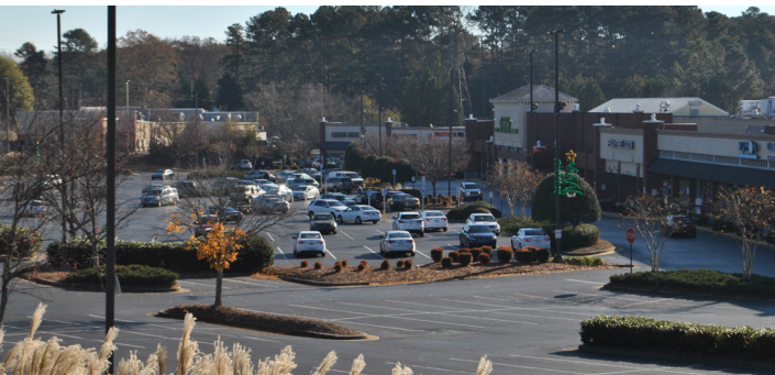
ABOVE: Current site conditions of the Duluth Station Shopping Center.
