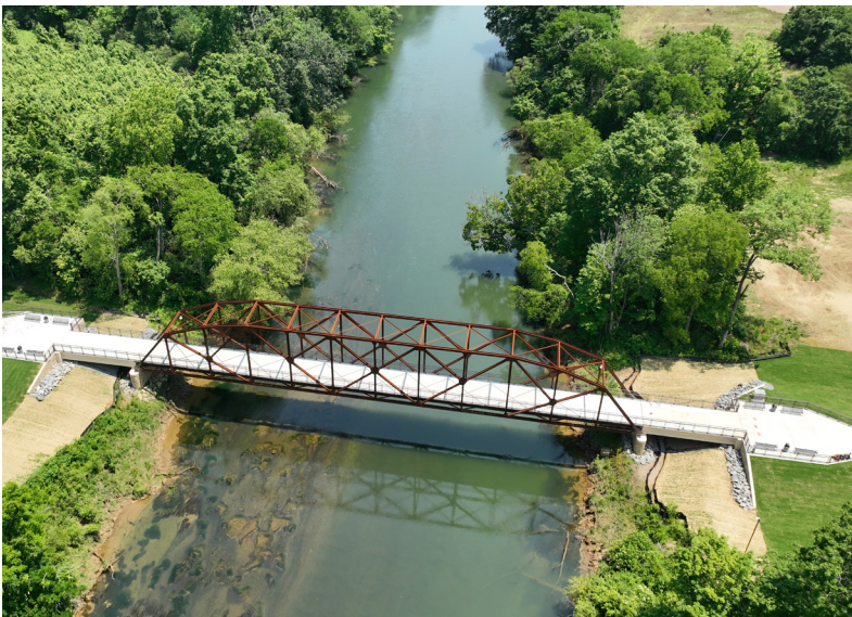
ABOVE: Reconstructed Rogers Bridge across the Chattahoochee River to Johns Creek.
