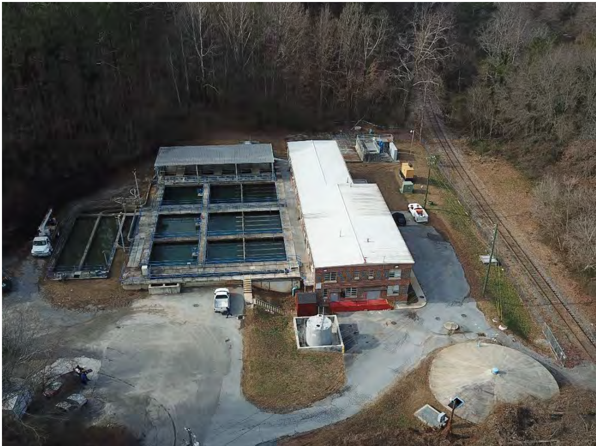
Canton Water Treatment Plant
