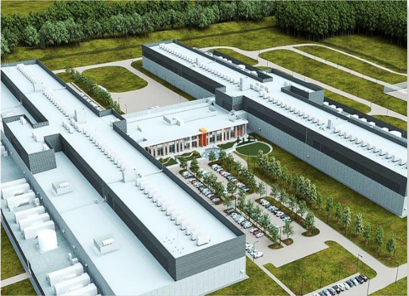
Source: Datacenterknowledge.com; Facebook Data Center in Huntsville, Alabama
