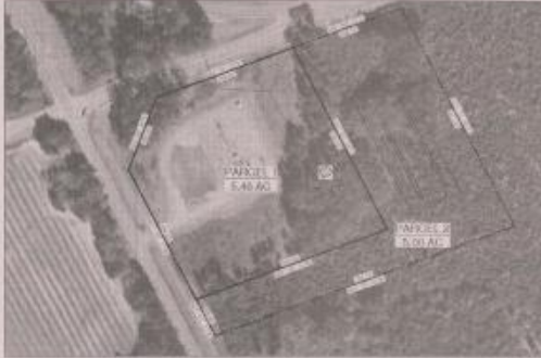
This aerial photo shows the new proposed site of the cryptocurrency mining operation within what "Parcel 2" Excelsior EMC obtained an option for this site after first proposing to place the facility inside "Parcel 1," which contains an existing power substation.
