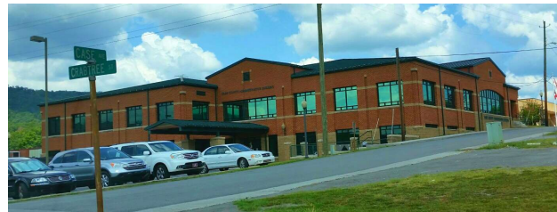
Figure 6. Dade County Administrative Building
