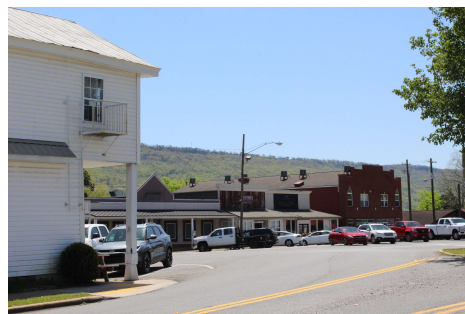
Figure 44. Local commercial establishments along Main Street on the downtown square
