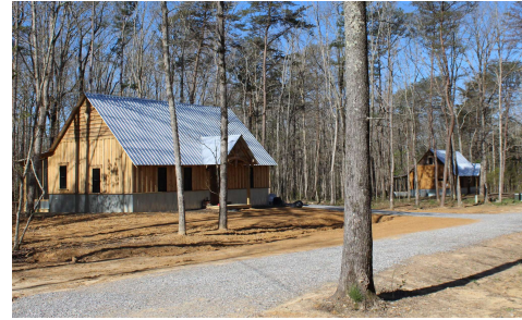
Figure 15. New Construction of housing in the New Salem Community Area
