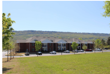
Figure 42. Multi-family residential on hwy 11
