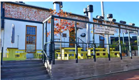
Industrial adaptive reuse project
