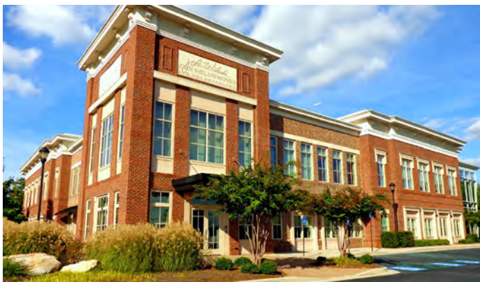
Office building on Atlanta Road
