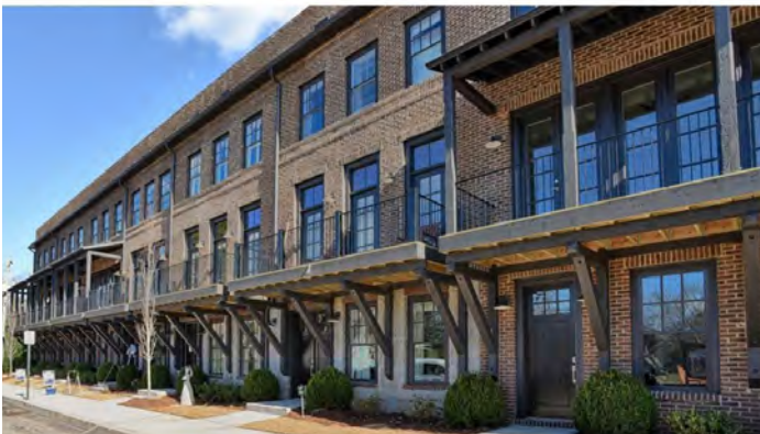
Multi-family residential in Old Fourth Ward in Atlanta
