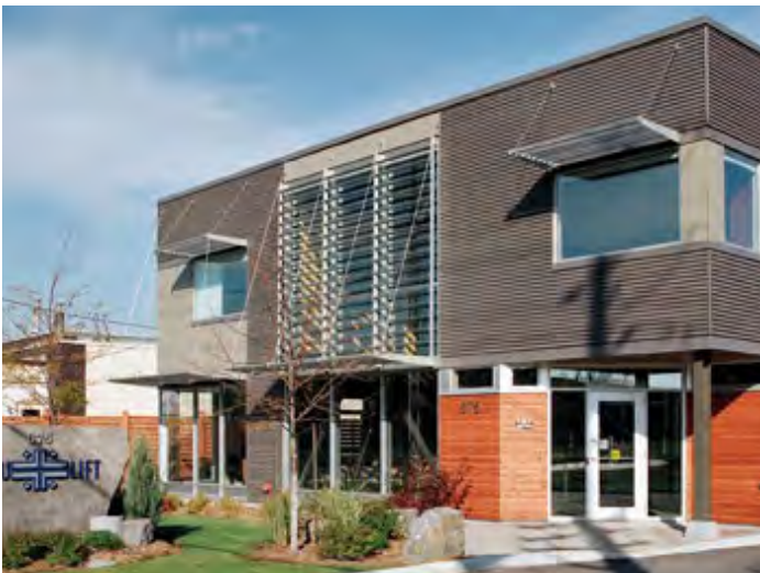
Sustainably designed light manufacturing facility
