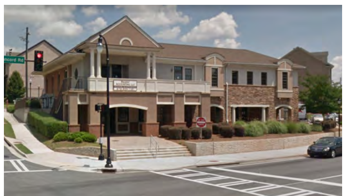
Office building on Concord Road
