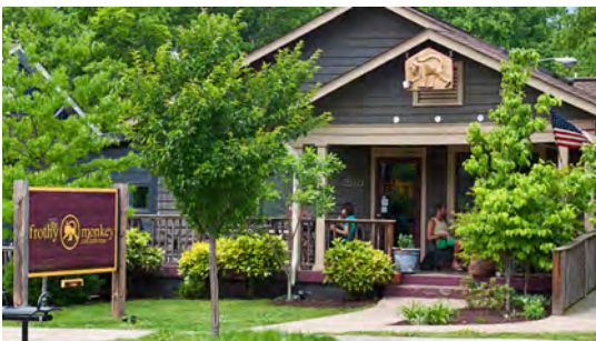
Home converted to business in Nashville, TN
