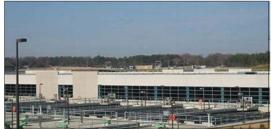
DeKalb County Water Treatment Plant
