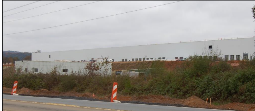
GE manufacturer in construction south of Appalachian Regional Port, Crandall.
