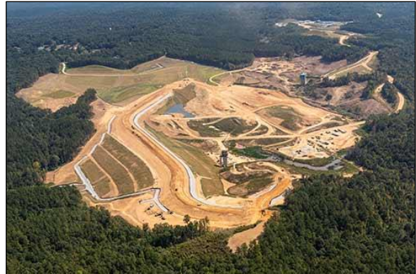
Paulding County Richland Creek Reservoir in construction.
