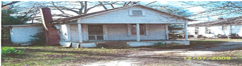
Substandard home on East Lee Street.
