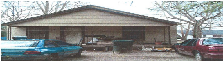
Substandard home and scattered debris on West Lillian Street.
