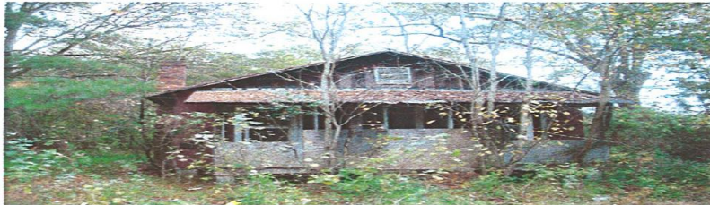
Abandoned dilapidated house along Salem Road.
