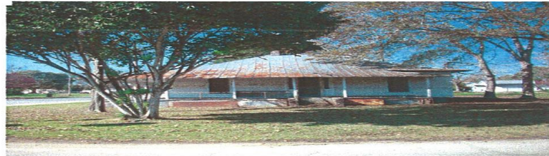
Substandard home on N. Terrell Street.
