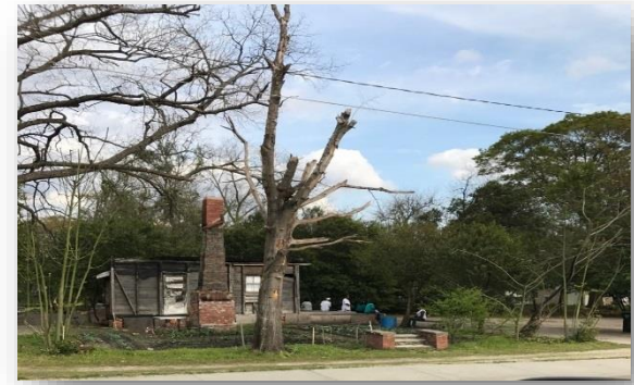
Dilapidated Structure in need of removal
