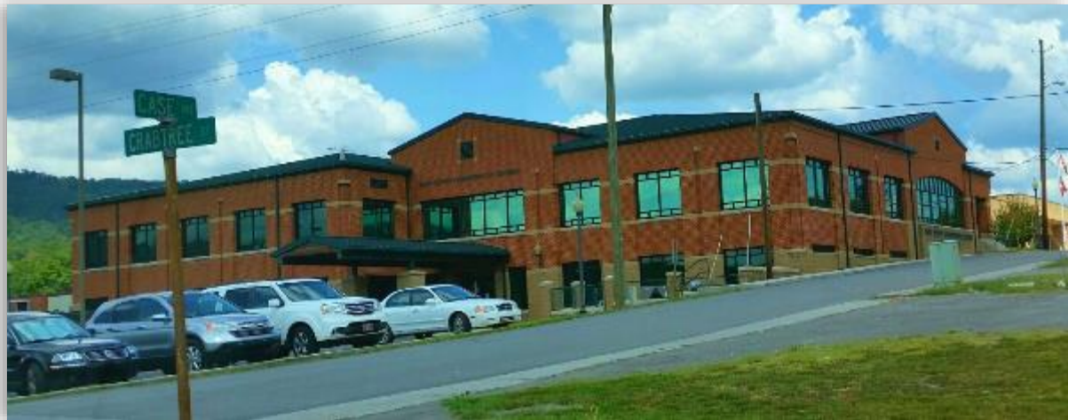
Figure 1 - Dade County Administrative Building
