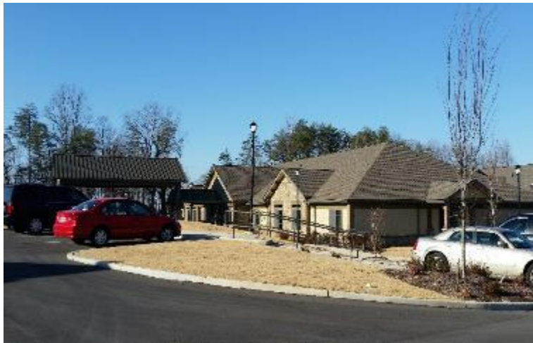
Figure 12 - Newly constructed Brow Wood, a planned community for active seniors
