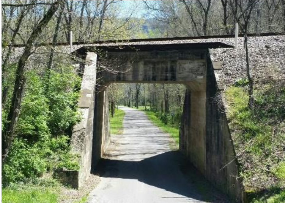
Figure 17 - Railroad overpass on Old Birmingham Hwy
