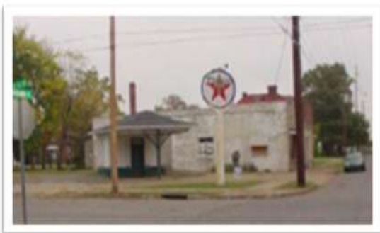
Building Rehab Before
