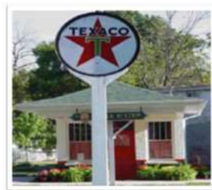
Building Rehab After
