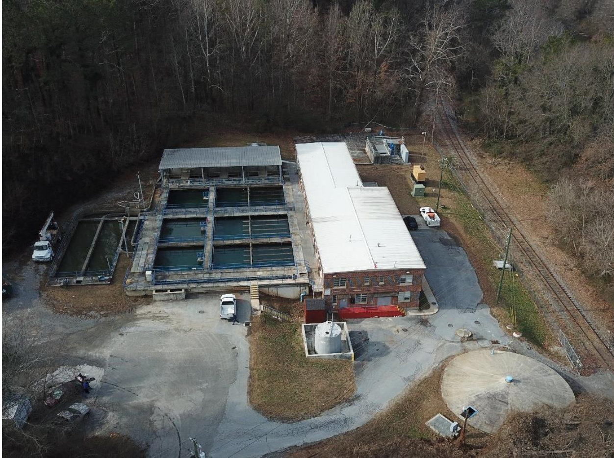
Canton Water Treatment Plant
