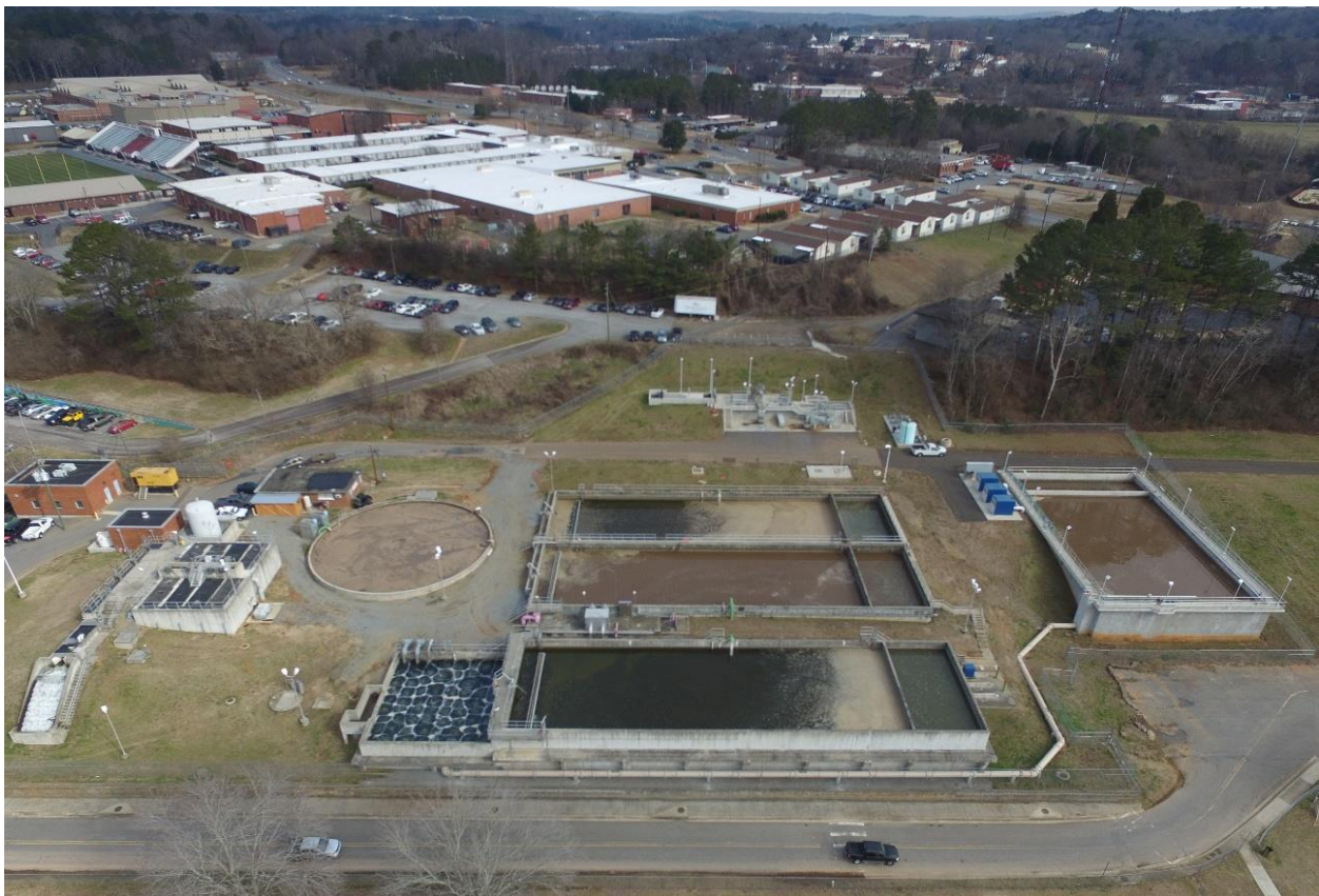
Canton Wastewater Treatment Plant
