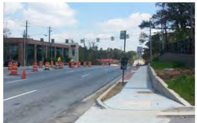
New sidewalk and street infrastructure along Buford Highway
