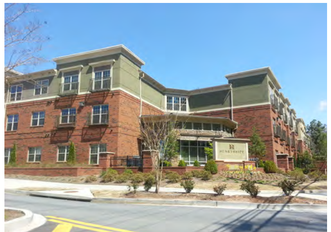
The Brookleigh development along Johnson Ferry Road has set a high standard for redevelopment.
