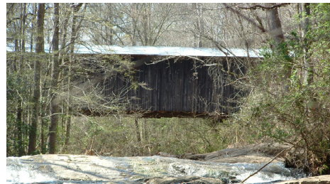
Elder Mill Bridge
