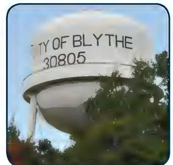
City of Blythe elevated water tank.
