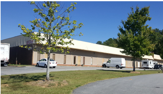
Warehouse on Martin Court
