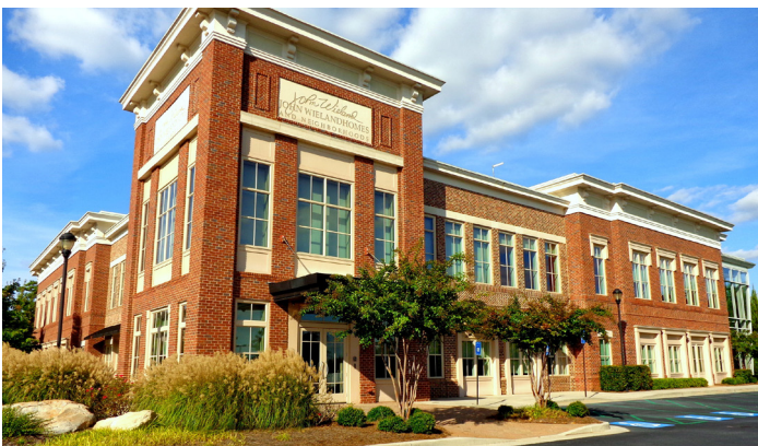
Office building on Atlanta Road
