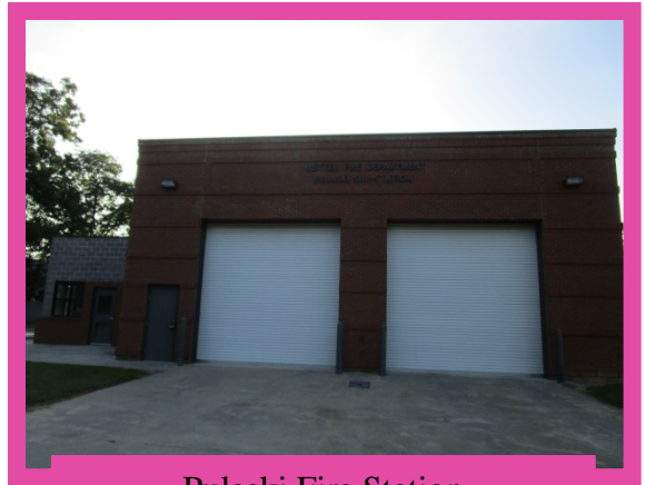
Pulaski Fire Station
