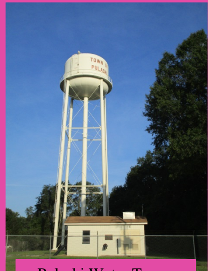
Pulaski Water Tower
