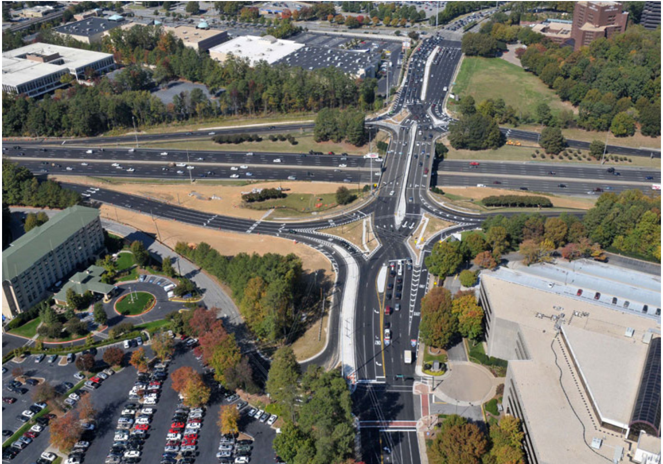
I-285 at Ashford Dunwoody Road is an example of some of the innovative infrastructure investments that region has implemented.
