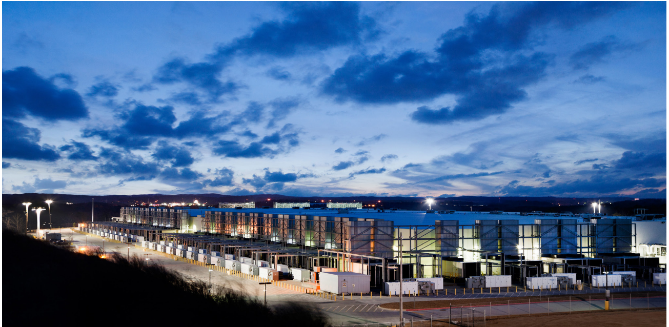
The Google Data Center in Douglas County (Image Courtesy of Google Inc.)
