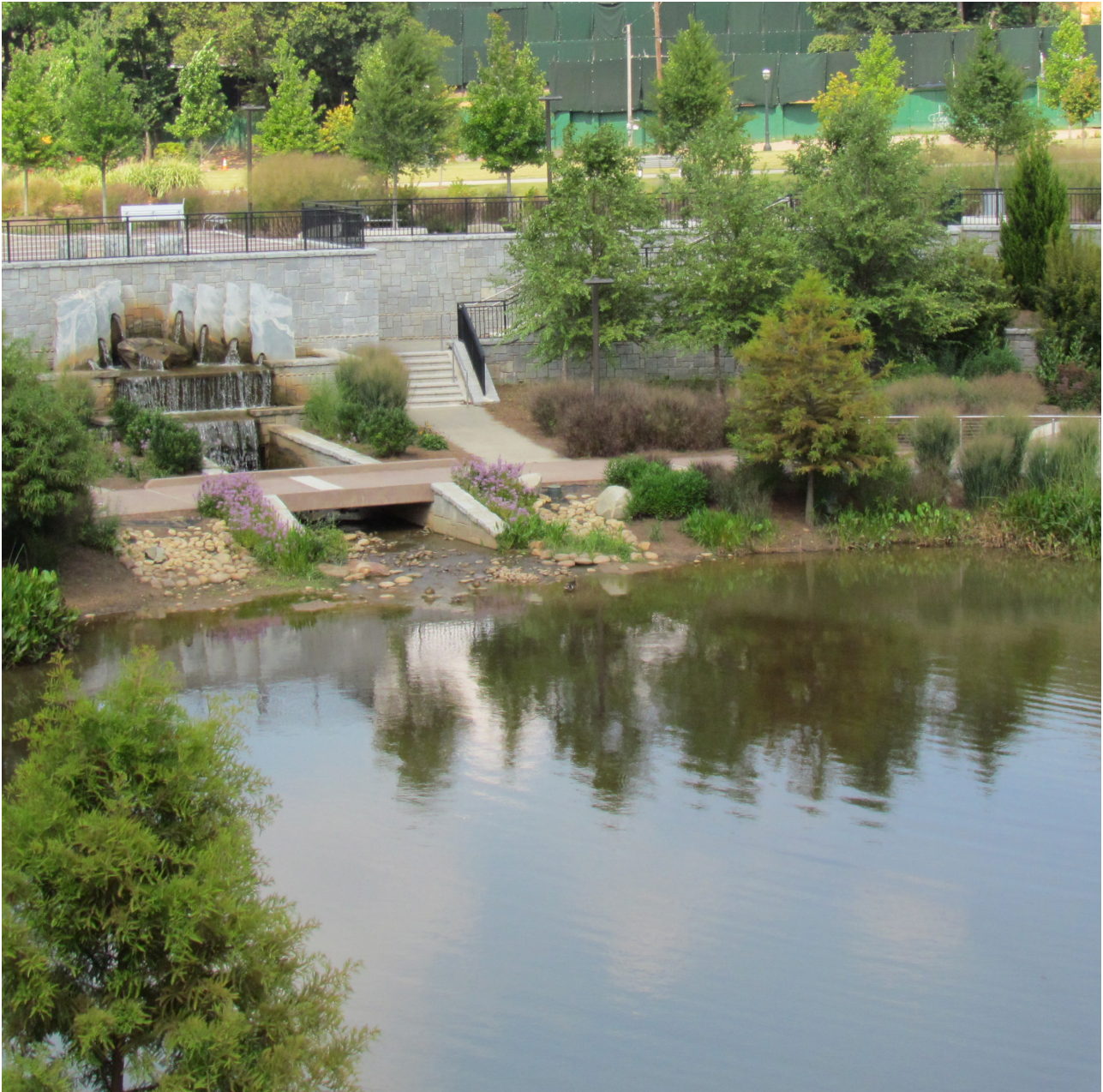
Old Fourth Ward Park in the City of Atlanta, is an example of using stormwater as a recreational amenity.
