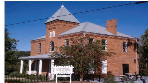
National Register Listed Historic Jail
