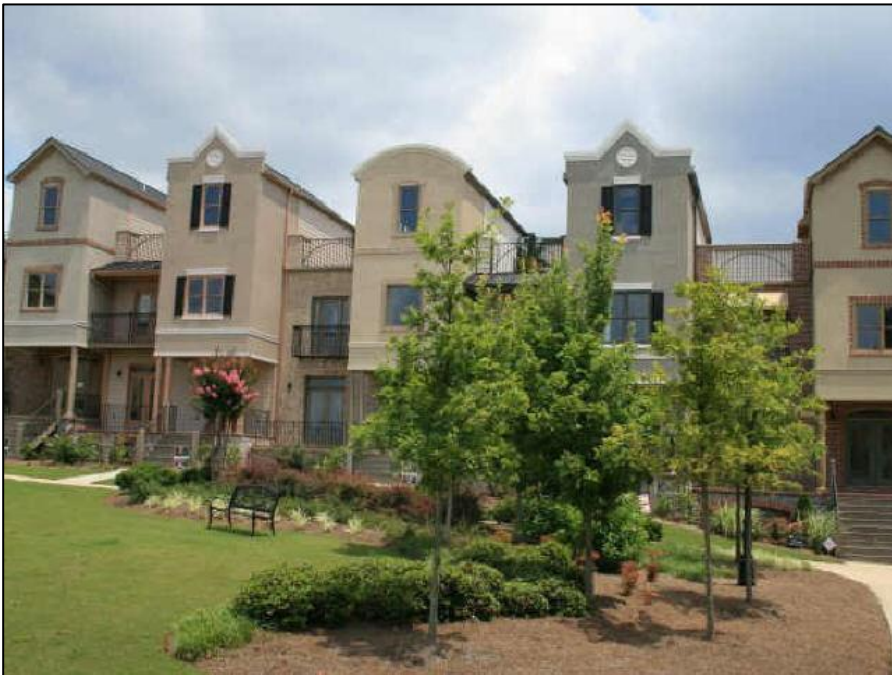
Towne Park Place townhomes located in Downtown Duluth
