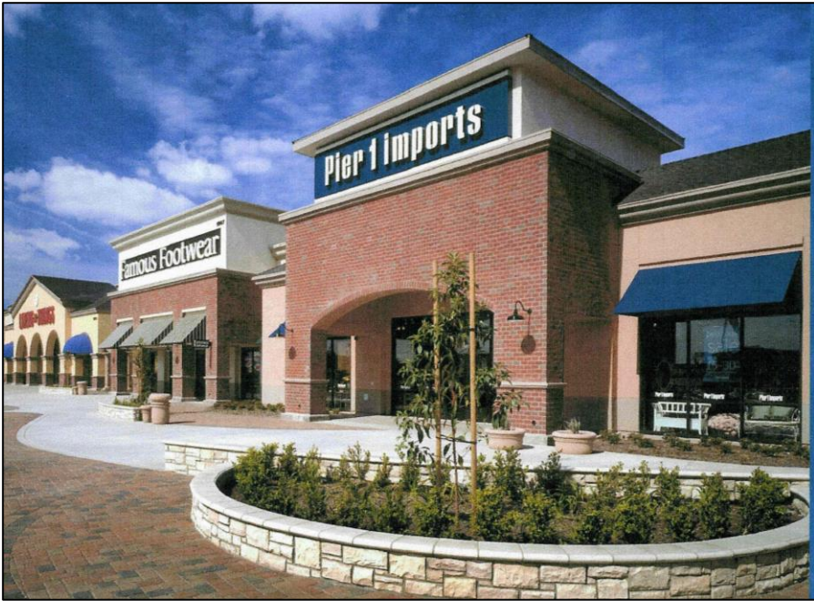
Well-articulated buildings with pitched roofs and canopies or awnings.
