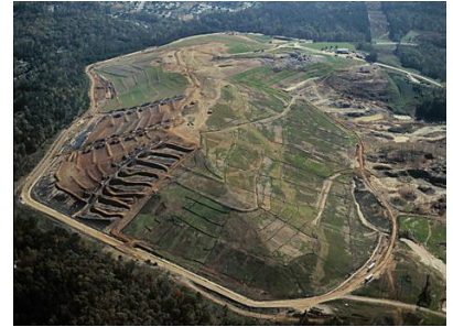
Aerial snapshot of the landfill
