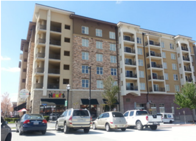
High density, multi-family housing with commercial on ground floor level, Town Brookhaven.
