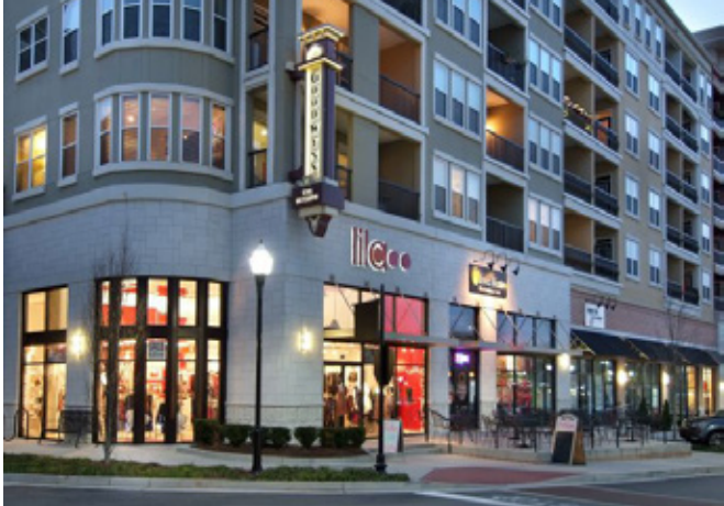
Mixed-use development with ground floor retail and residential above, like that shown above in Town Brookhaven, is desired for this area to balance the land use mix, which is currently dominated by large-scale office development. Photo Credit: townbrookhaven.net
