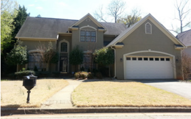
Many neighborhoods in this character area built in the 1980's and 1990's lack sidewalks.
