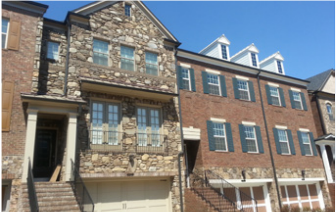
The mix of housing options at the Brookleigh development on Johnson Ferry Road is a good model for future housing in Brookhaven
