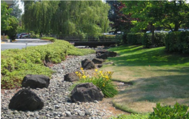
Encouraging bioswales and other ecological design solutions can help promote positive stormwater management
