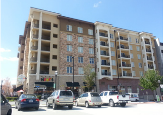
Town Brookhaven is a large-scale mixed-use development along Peachtree Road.
