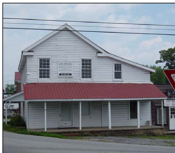
Figure 1-1: Historic building in Dawsonville
