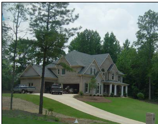
Planned Community residence in Chestatee development in Dawson County
