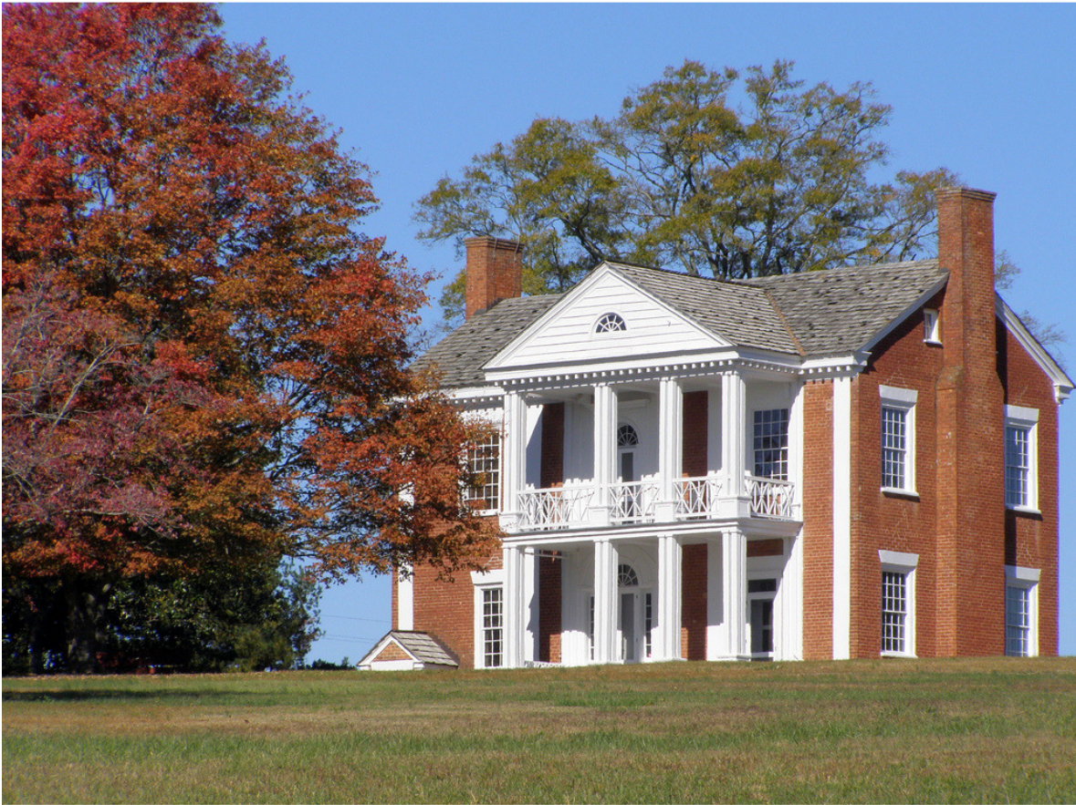
The Vann House
