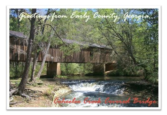
The bridge uses steel rods as tension members in its truss design. The result is similar to a queen post or Warren truss. The angled rod design makes the bridge unique not only in Georgia but the entire U.S. Citizens of Early County undertook a restoration project in 1984 to stabilize and repair the bridge, which remains in sound structural condition today.
