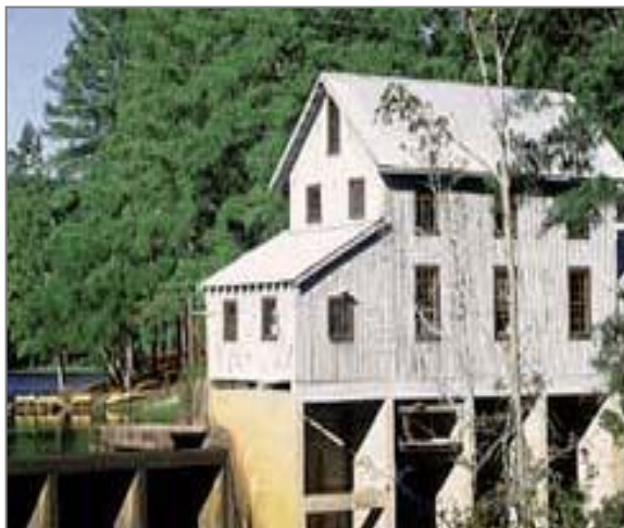
Picture 4: Water-powered grist mill at Hamburg SP
