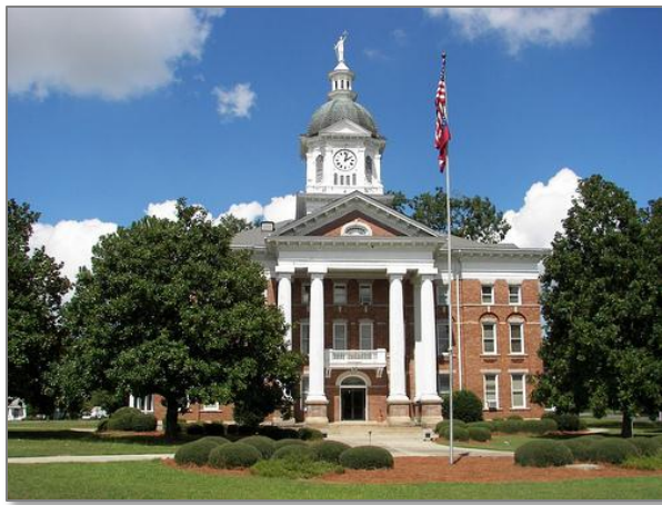
Picture 34: Jenkins County Courthouse
