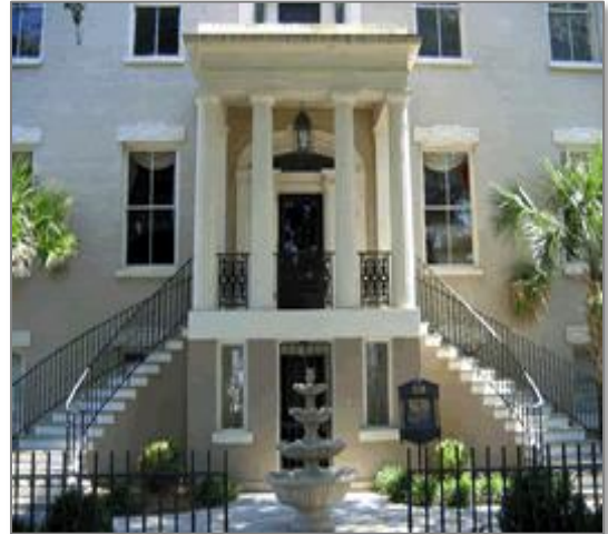
Picture 32: Phinzy House located in the Historic Augusta District
