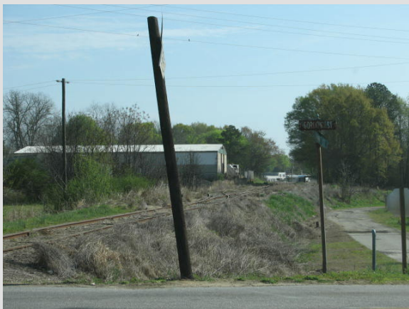
The Rail Head Business Area includes some active businesses, but is also characterized by multiple, small, unused sites; and, is split by a number of short rail tracks which terminate in the area.
