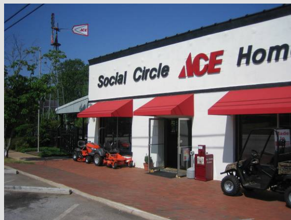
Central business districts across rural Georgia continue to be viable centers of commerce – as illustrated by this renovated hardware store in Social Circle, Georgia.
