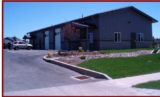
New Light Industrial building with landscaping, sidewalks, and quality materials
