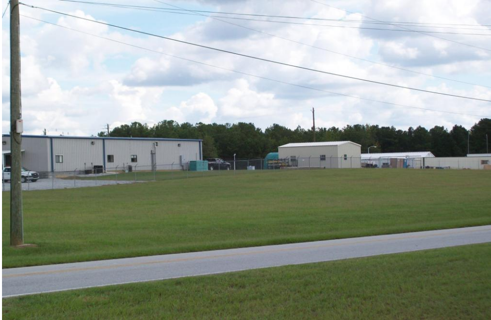
Natural gas storage facility, McKenzie Road.
