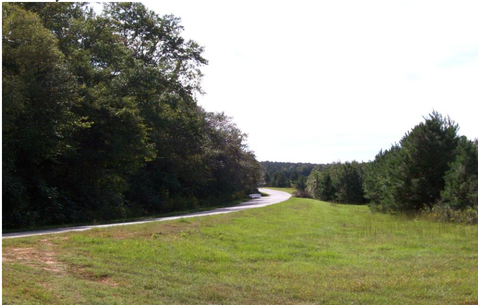
City Pond Road near reservoir.
