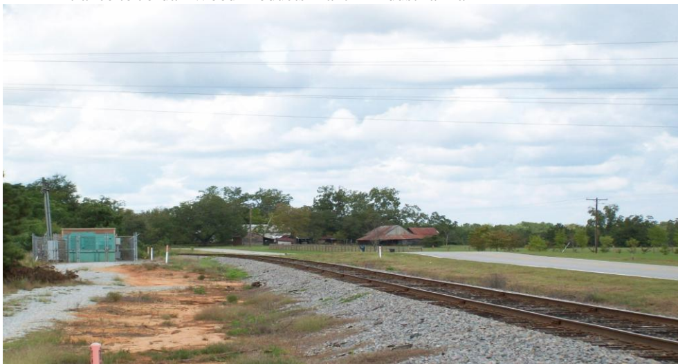
Railroad tracks and Old Milner Rd separating Industrial Park from farm land.
