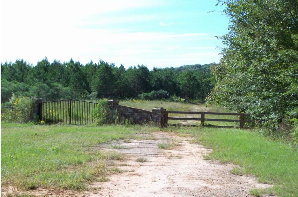
Entrance to reserved area north of reservoir.
