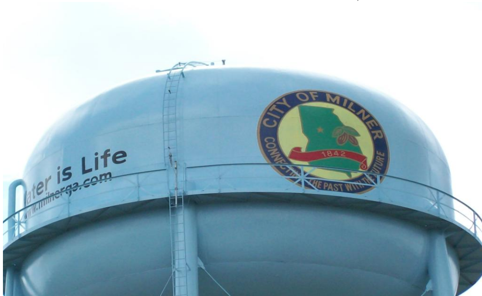
Mid-town Water Tank, Milner
