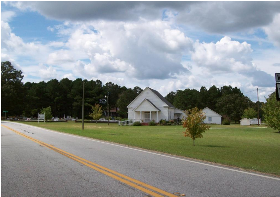
Ebenezer UMC at intersection of Hwys 18 & 109.
