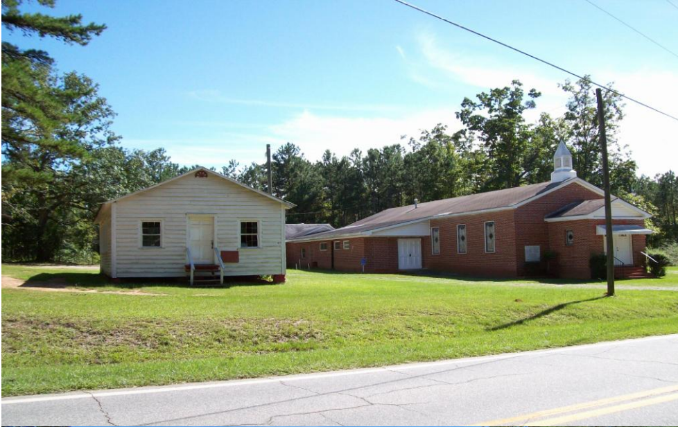
Unionville UMC on High Falls Park Road.
