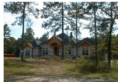
New house under construction.
