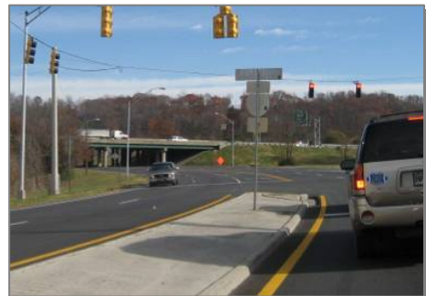
Interstate Gateway District
