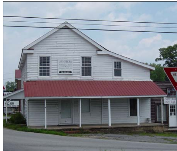
Figure 2-1: Historic building in Dawsonville
