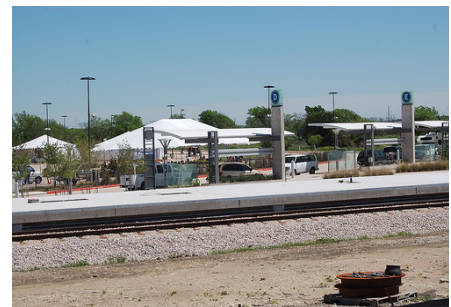
Leander, TX Commuter Station
