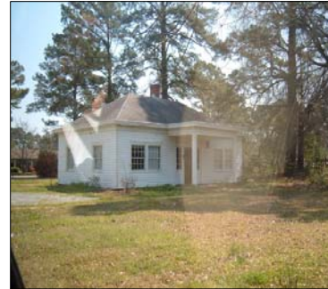
The Pay Station Building
