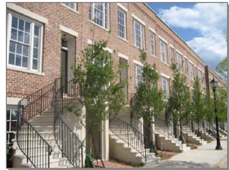
A wider range of housing types in limited areas of the county, such as attached townhomes shown above integrated into a larger mixed use neighborhood, is needed in order to meet the anticipated demand of changing demographics in Banks County
