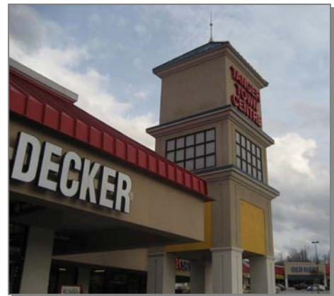
Existing commercial development in Banks Crossing's Tanger Outlet
