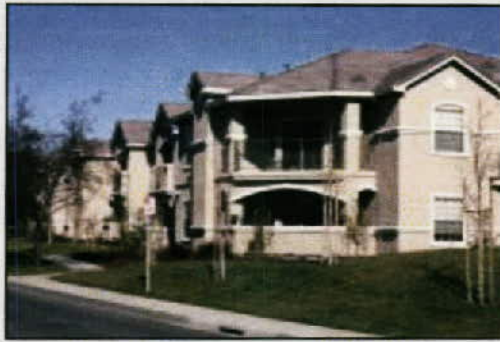
New infill residential development should be compatible with the scale and density of existing development
