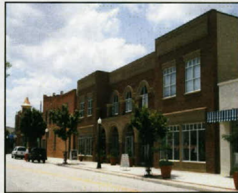
New commercial development close to the street improves visibility and creates a pedestrian-friendly shopping environment.
