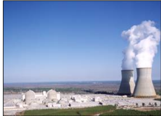
Energy Production District – Plant Vogtle
