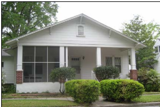
Housing conditions in the Town Neighborhood Revitalization area in northwest Waynesboro vary from good (above) to poor condition(below).
