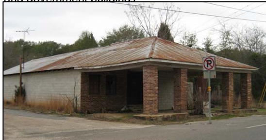
Keysville Town Center includes redevelopment opportunities, such as this building on SR 88
