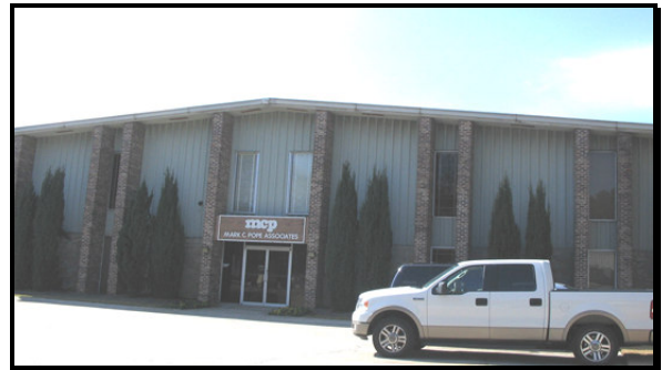
Industrial Park with Landscaping
