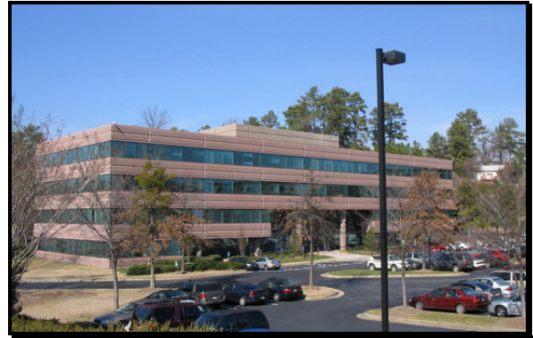
Office Building - Four Story
