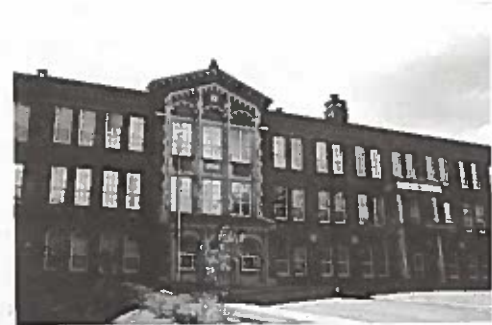
Brown Middle School (former high school) was built in 1923. The Romanesque Revival-style school was named in honor of Joseph E. Brown, governor of Georgia from 1857-1865. This community landmark building in the West End Historic District was one of the first schools in Atlanta to be integrated in 1961. Photo by Jeanne Cyriaque
