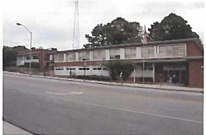
Beacon Elementary School and the City of Decatur received a Historic Preservation Fund grant through the Historic Preservation Division in 2010 that funded a conditions assessment by Rutledge Alcock Architects. Photo by Jeanne Cyriaque
