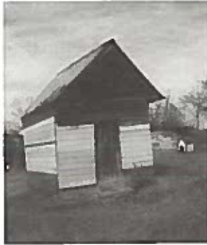
The smokehouse on the Morgan farm features a raised-seam, metal roof, and a log foundation. It was built circa 1890 and used until 1993. HPD File Photo
