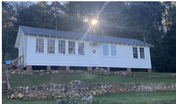
Before and after: The Fairview School project in Floyd County rehabilitated as of 2022. Photos courtesy of The Fairview/Brown E.S. School Foundation.
