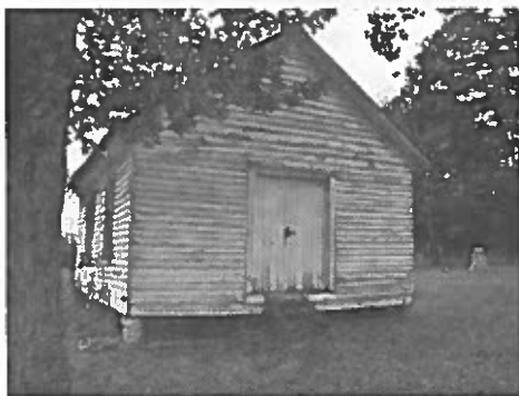
The Cherry Grove School is located next to the Cherry Grove Baptist Church and Cemetery in Wilkes County. It is a rare, one-room, wood frame building and is distinguished by its stone pier foundation.
