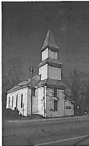
Freed slaves built Jackson Chapel A.M.E. Church in 1867 to serve the African American community called Wylieville in Washington. The church is a community landmark building in the Washington Historic District.
