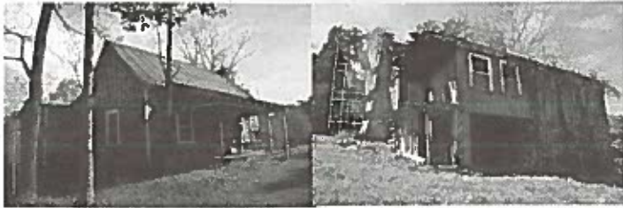
The slave cabin's original appearance was modified by adding interior rooms, windows and a front porch. These deteriorated elements were removed to restore the slave cabin to its original size. Photo by Jeanne Cyriaque
