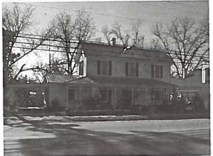
Dr. Sessoms constructed this two-story, Folk Victorian style I-house around 1890. He built the home for his family and medical practice. His office was located on the first floor with a separate, covered entrance for patients.
