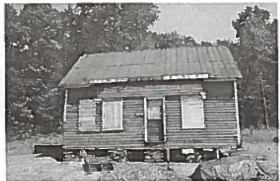
This photo shows the slave cabin resting on the original rock piers in its new home at the Nacoochee Valley African American Heritage Site & Nature Preserve. Stone mason David Vandiver will reassemble the rock chimney and hearth. Photo by Jeanne Cyriaque
