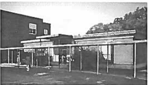
The Risley Alumni Association are the stewards for this building on the campus. It is located between Colored Memorial School and the former Risley High School. Photo by Linda Cooks
