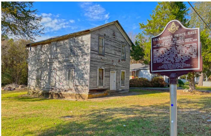
Chickamauga Masonic Lodge No. 221 Photo Courtesy of The Georgia Trust
