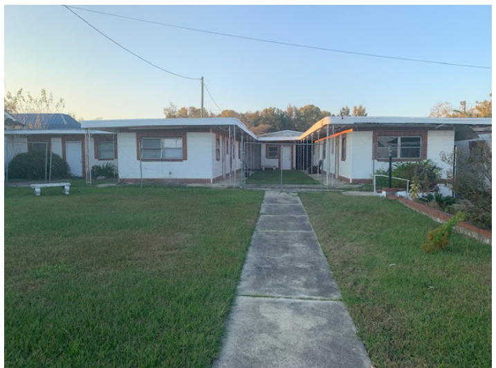
The Dudley Hotel Photo Courtesy of The Georgia Trust
