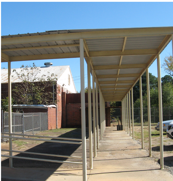
Walkway leads to Gym (foreground) built in 1958. Credit: Melissa Jest/Georgia Historic Preservation Division
