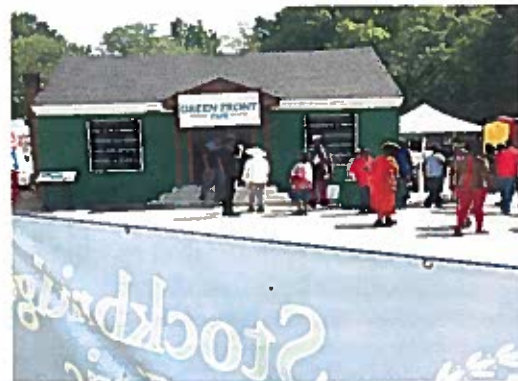
The Green Front Café is currently under renovation.
