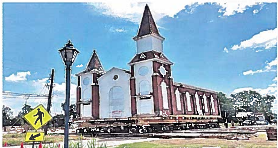
The relocation of Mother Trinity took three days. Courtesy of Augusta Canal Authority
