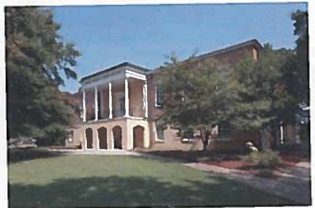
The Warren A. Candler Memorial Library was completed in 1947. The building was repurposed for use as administrative offices and special events in 1991. Photo by Charlie Miller
