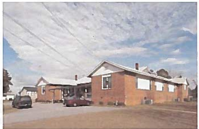
The 1926 Rosenwald School lies adjacent to the 1959 equalization school complex. This building is adaptively used today as a community center.
