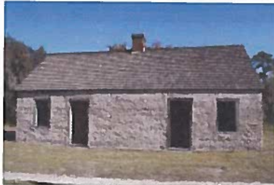
Tabby cabin #2 features dual front entrances and a central fireplace. Photo by Jeanne Cyriaque
